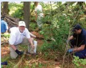
Williams Woods Trail Work – Charlotte
