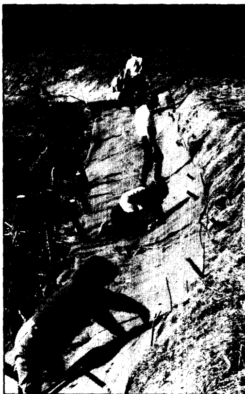
Volunteers install an erosion control mat at the 1824 House Inn streambank stabilization site. Photo by Kinny Connell
