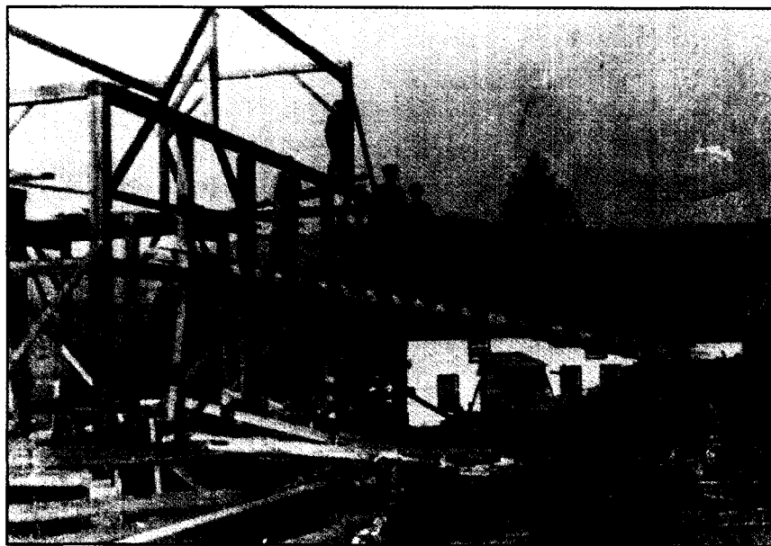
Raising the high bank barn on the McLaughlin farm, 1923. This barn was disassembled in Waitsfield, moved to Fayston, then reassembled piece by piece.
